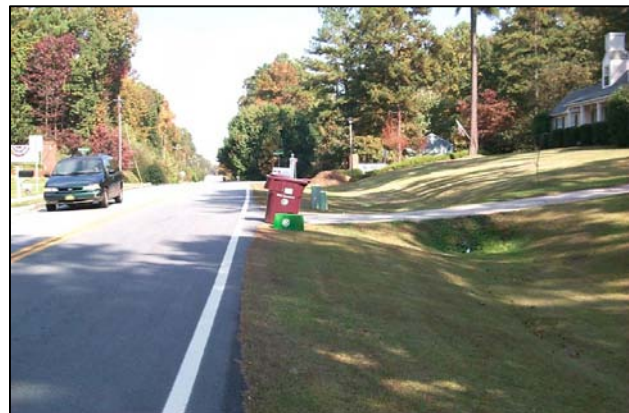
Figure 4.2-21 Using Vegetated Swales Instead of Curb and Gutter
