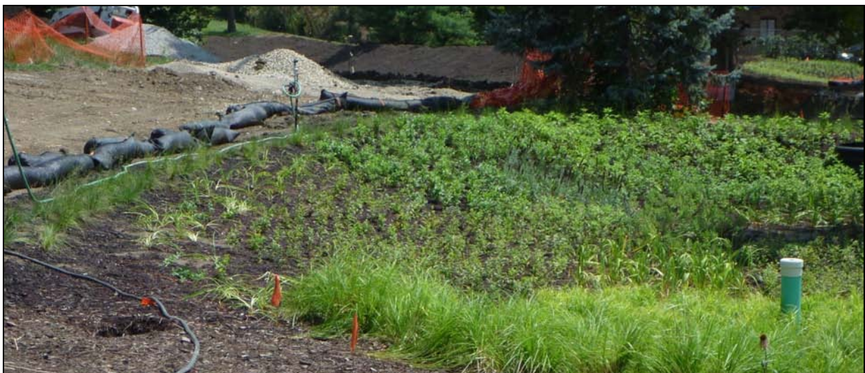
Figure 7.2-1 Erosion prevention and sediment control measures (sand bags) used to prevent sediment from flowing into rain garden.
