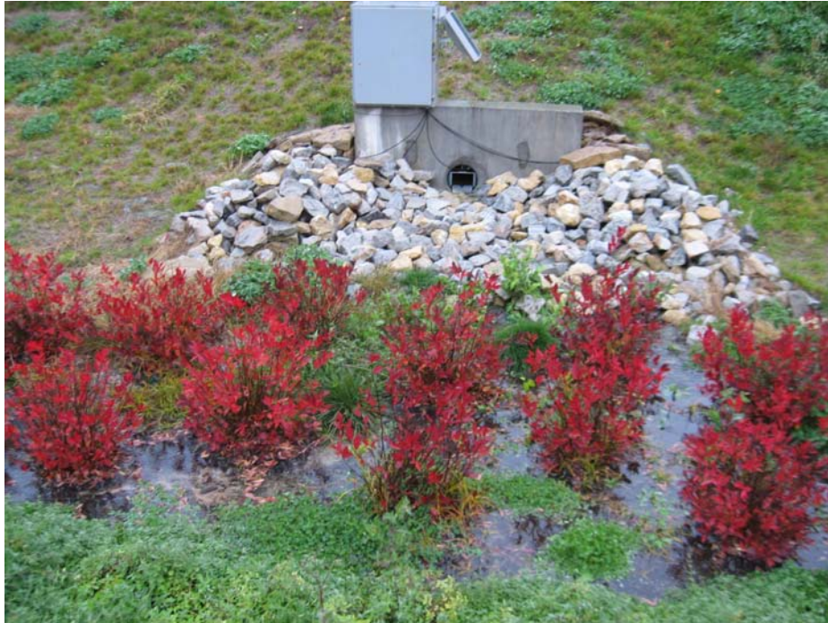
Figure 7.2-3 Energy dissipation (rip-rap) at point of discharge into bioretention basin.
