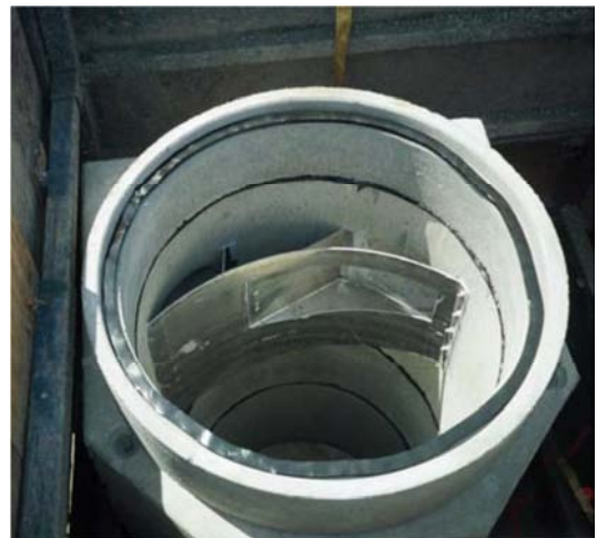
Hydrodynamic Separator; Contech Stormwater Solutions http://www.contech-cpi.com/Products/Stormwater-Management.aspx
