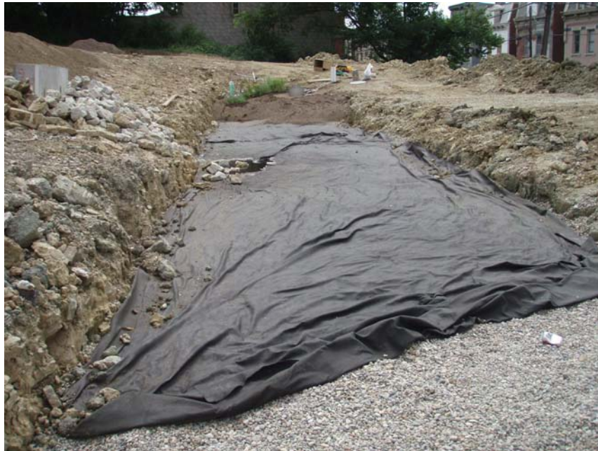
Figure 7.2-2 Installation of non-woven geotextile filter fabric between planting media and drain rock.
