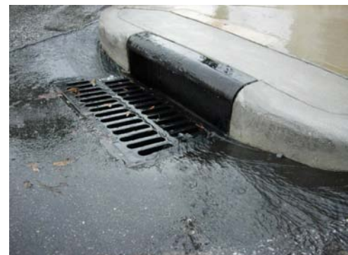
Figure 2.1-2 Impervious Cover Increases Runoff Peak Flows and Volumes While Reducing Recharge
